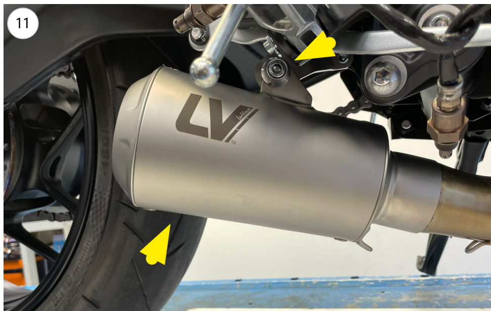
install the muffler
